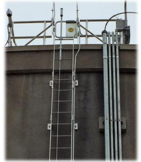
**Swing Gate for a Vertical Ladder on an Elevated Surface**
