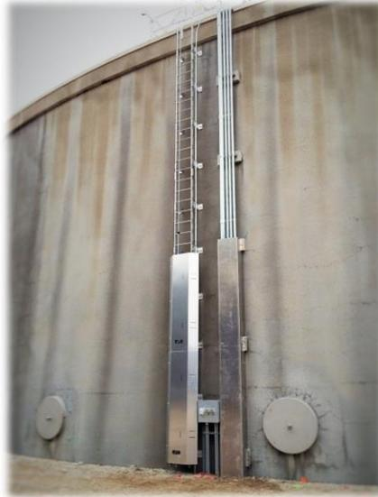
**Vertical Ladder Safety System on Water Tower**
