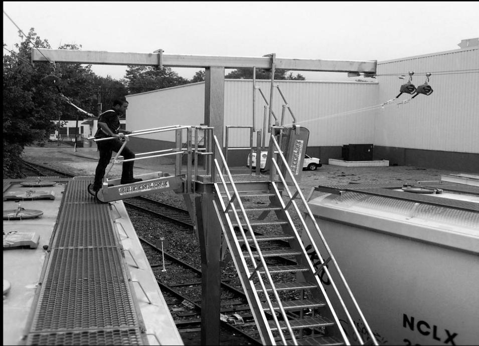
ABOVE PHOTO: END ANCHOR SUPPORT WITH DROP DOWN GANGWAYS FOR SAFE ACCESS TO THE TOP OF RAILCARS ON PARALLEL TRACKS.
